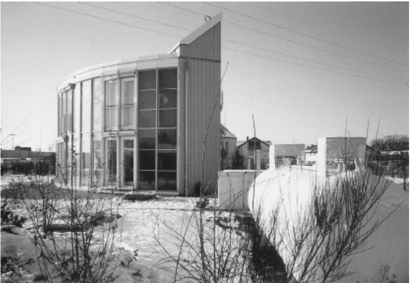
The solar hydrogen house built by the Fraunhofer Institute for Solar Energy Systems in Freiburg, Germany. The hydrogen tank is in right foreground. (courtesy of Fraunhofer Institute for Solar Energy Systems)
